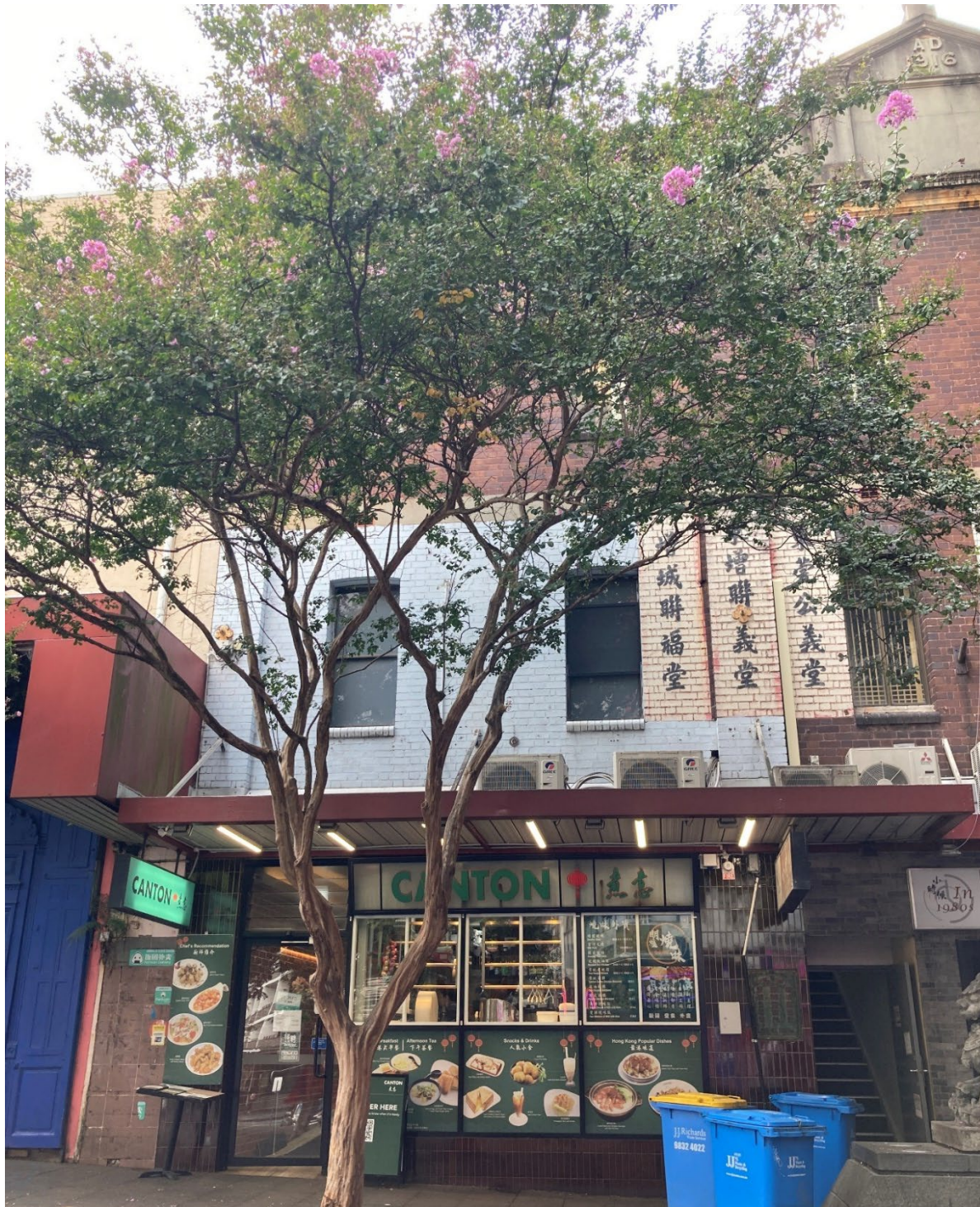
Figure 26. View of 50 Dixon Street. Source: HAA, 2024.
