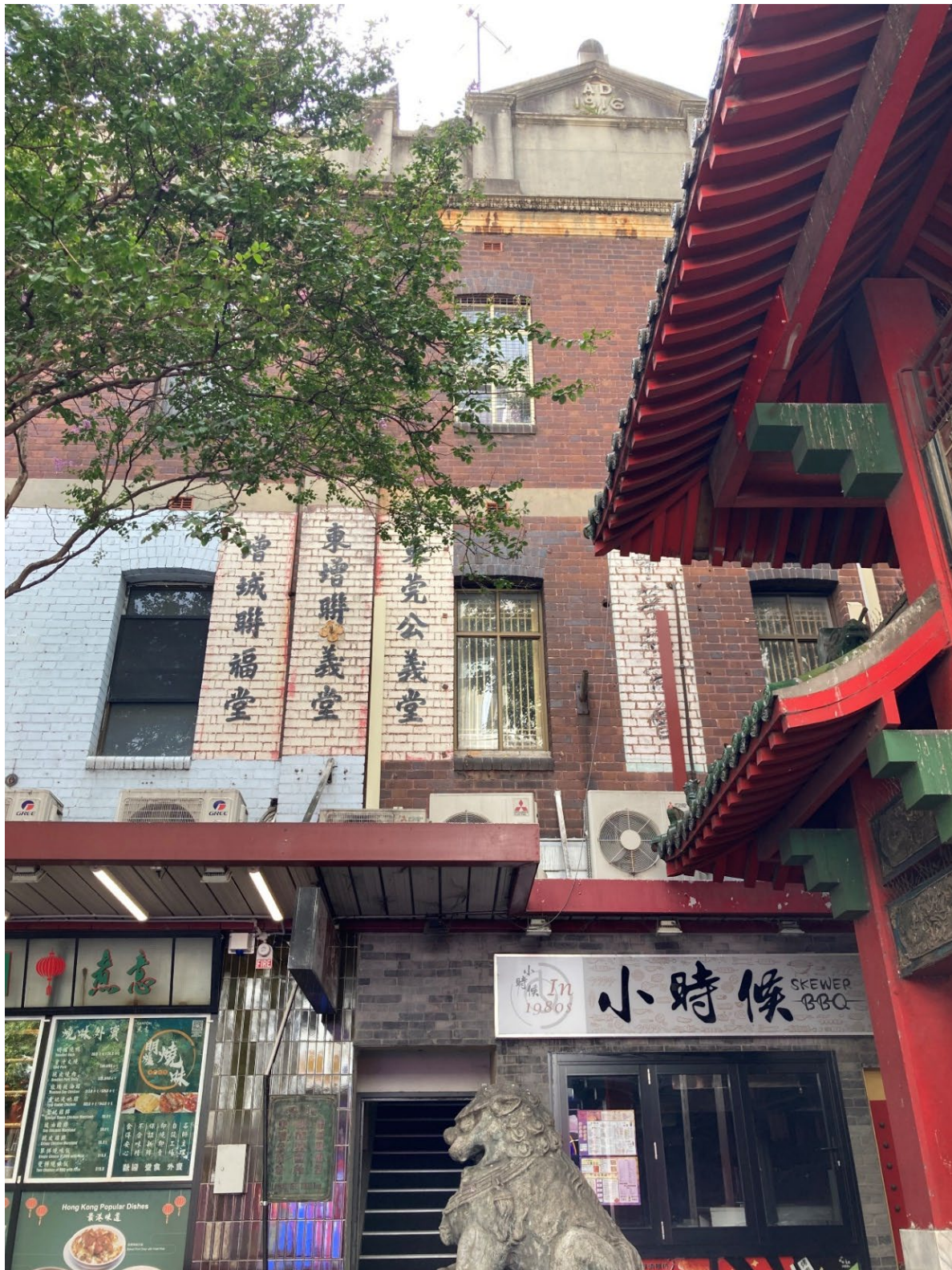
Figure 28. View of 52 Dixon Street. Source: HAA, 2024.
