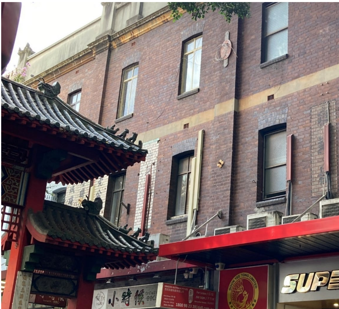
Figure 29. View of 52 Dixon Street. Source: HAA, 2024.
