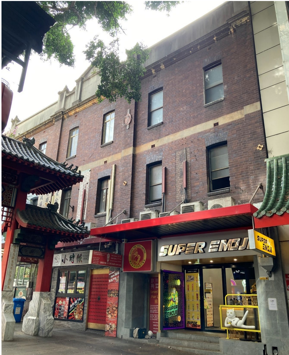
Figure 24. External view of 50-54 Dixon Street. Source: HAA, 2024.
